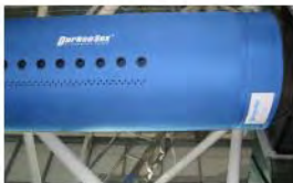
Generally straight duct suggested to be less than 9m/s
