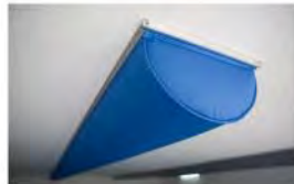
large half round duct suggested to be less than 8m/s
