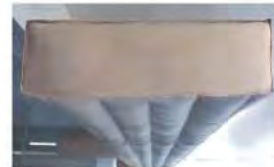
rectangle duct suggested to be less than 8m/s
