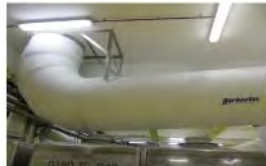
elbow suggested to be less than 8m/s
